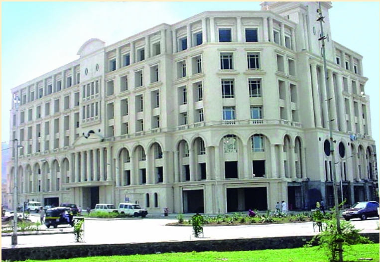
MIXED-USE DEVELOPMENT: The IT park at the Hiranandani complex in Mumbai is a mixed-use project
