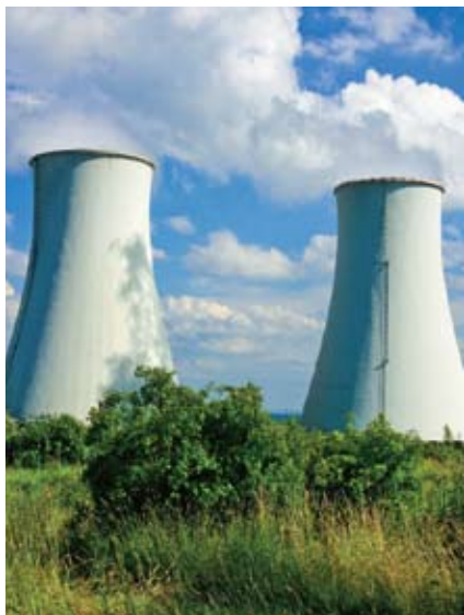
TOWERING GROWTH: With its strong engineering base, Alstom is able to contribute significantly to India's power sector
